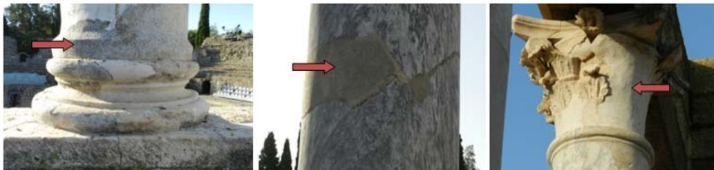
**Fig. 3.** Restoration mortars used in different periods for the structural consolidation of the Front stage in the Roman Theater of Merida (Photos by Natalia Perez)
