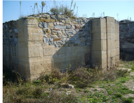
Fig. 2. Consolidation-restoration of the fortress walls.
