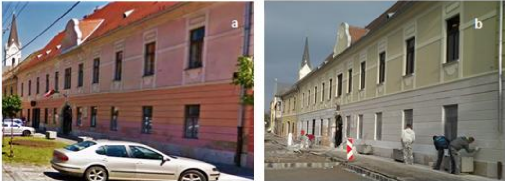
Fig. 1. Renovation of the buildings on Kossuth Lajos Street, St. Gy r, Gyor-Moson-Sopron: a – picture from Google Earth, May 2014; b - personal photo, November, 2014.
