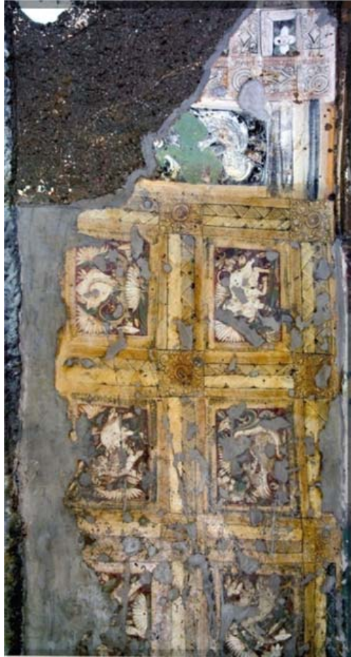
Fig. 1. Painted mortar of Cave no.19, Ajanta applied with shellac varnish
